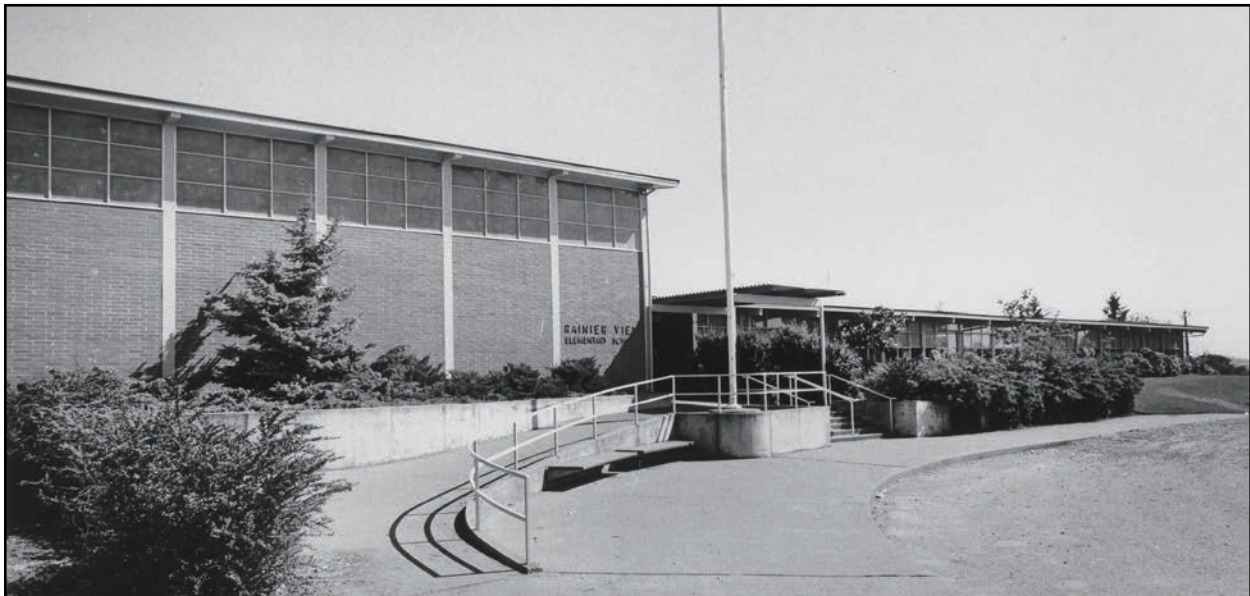
Figure 20 • Rainier View Elementary (1961, Durham, Anderson & Freed)
