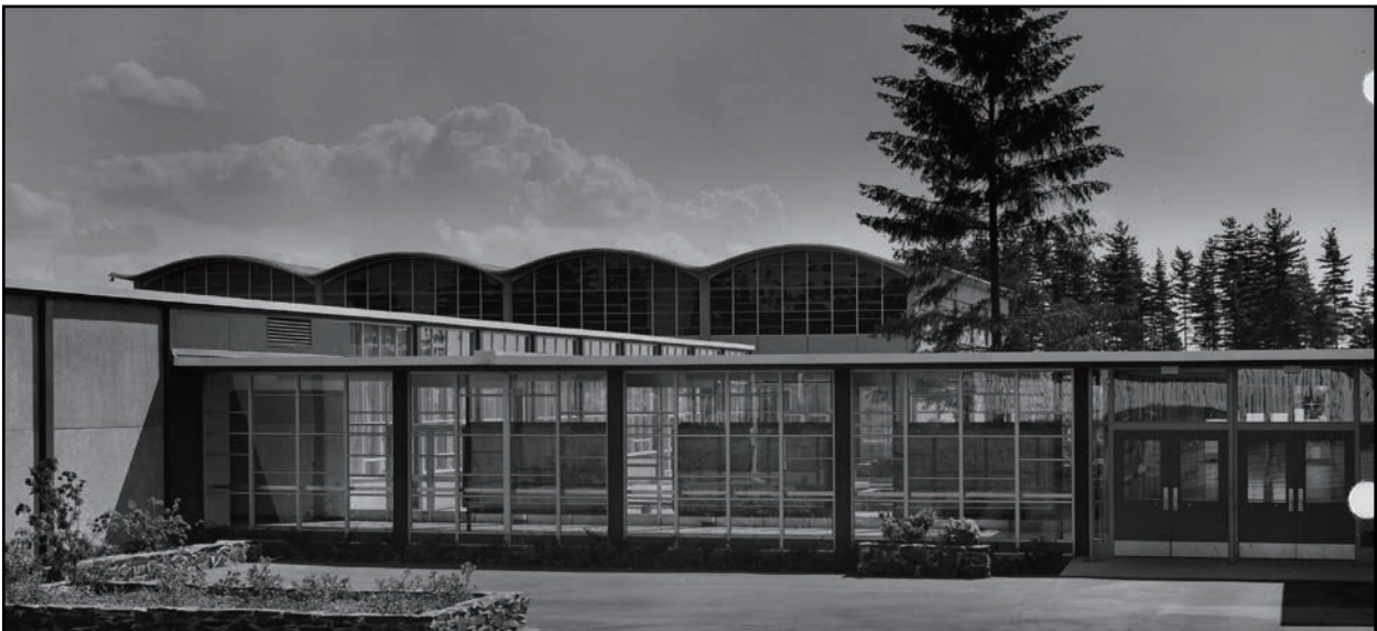
Figure 34 • Ingraham High School (1959, Naramore, Bain, Brady, & Johnson, partial City of Seattle Landmark)
